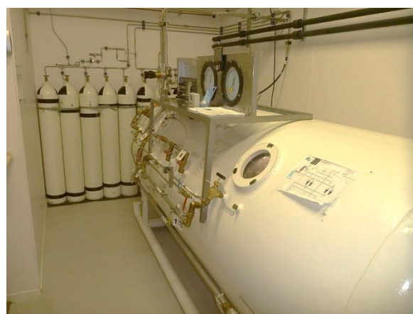
Decompression chamber with air banks and the extra line (Photo: Svein Harald Sønderland)
