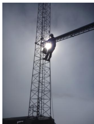
NILU engineer Are Bäcklund about to install a new air inlet for the Medusa instrument. Photo: NILU
